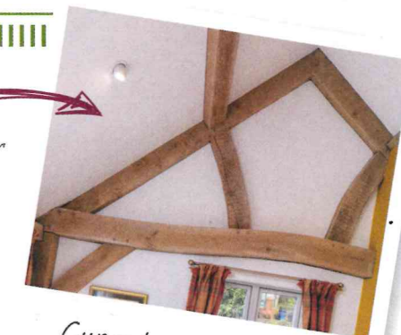
Curved wood beams
